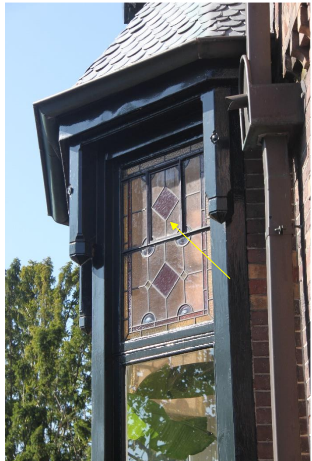
foto 19. Detail glas in lood bovenramen met ventilatieopening (origineel) in erker, 2021, [redacted]
